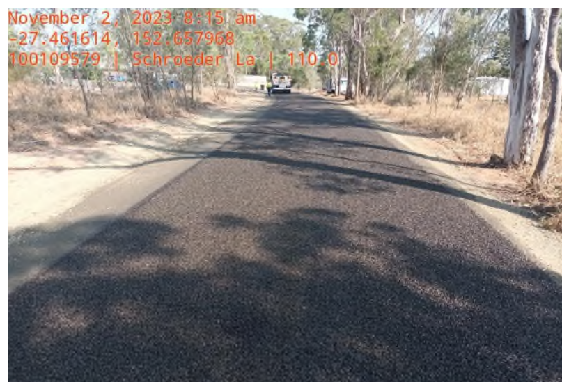
Schroeder Lane, Fernvale – upgrade from gravel road to bitumen, and seal intersection with Fairney View Fernvale Road
