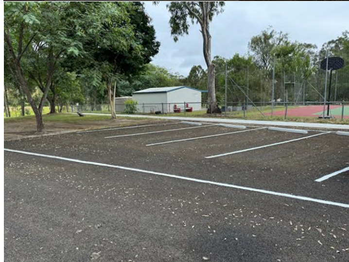
Linville State School, Wells Street, Linville – new footpath, reseal of parking area with linemarking and wheel-stops. Funding: Queensland Government Transport Infrastructure Development Scheme
