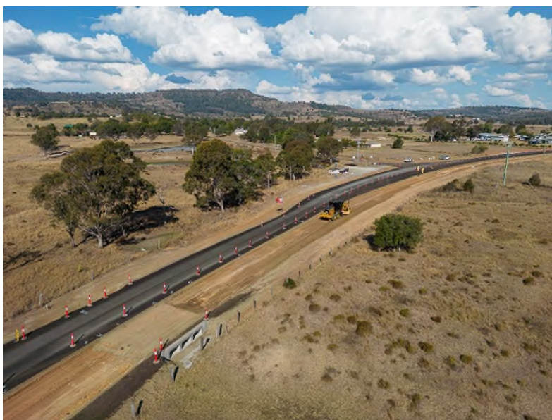
Lowood Minden Road (Litzows to Lukritz) – road widening, pavement stabilisation, sealed shoulders, new culverts and pipes. Funding: Australia Government Heavy Vehicle Safety and Productivity Program
