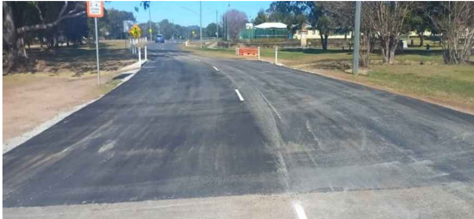
Cressbrook Street, Toogoolawah – culvert replacement and asphalt overlay.
