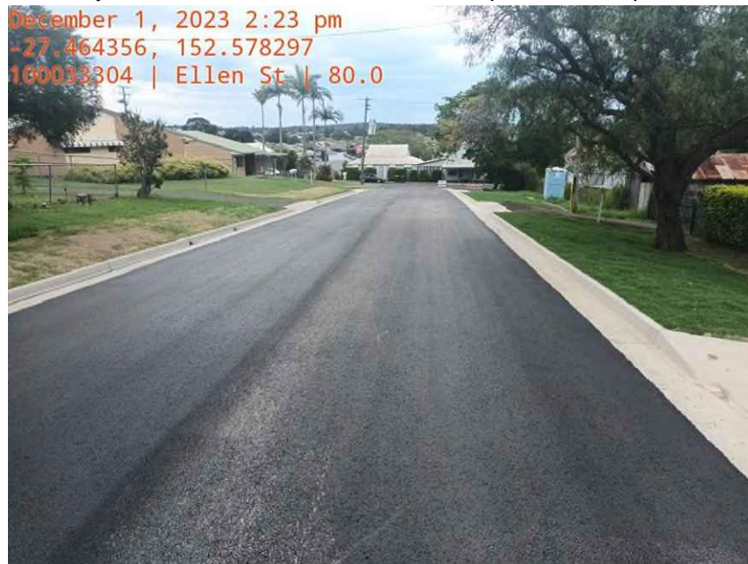
Ellen Street, Lowood – kerb & channel and two-coat seal
