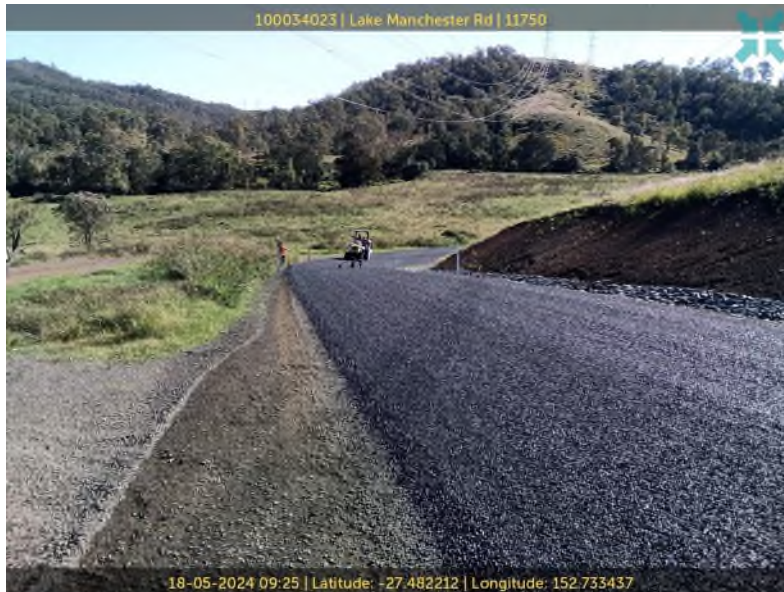
Waverley and Sheppards Road, Lake Manchester – six metre, two-coat bitumen seal Funding: Australian Government Black Summer Bushfire Recovery program
