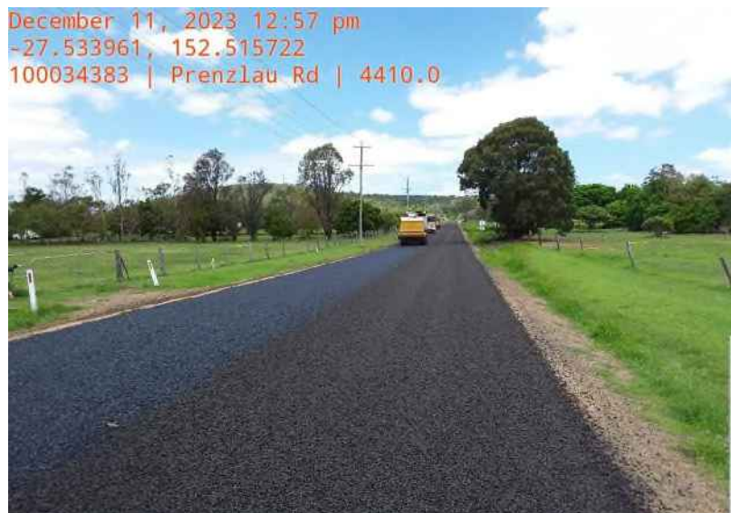
Prenzlau Road, Prenzlau – pavement reconstruction of Prenzlau Road, and two-coat seal;
