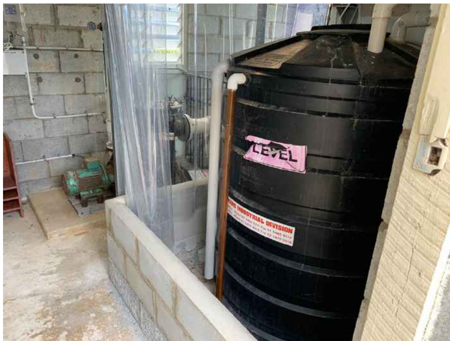
Figure 11: Chlorine storage tank in bund
