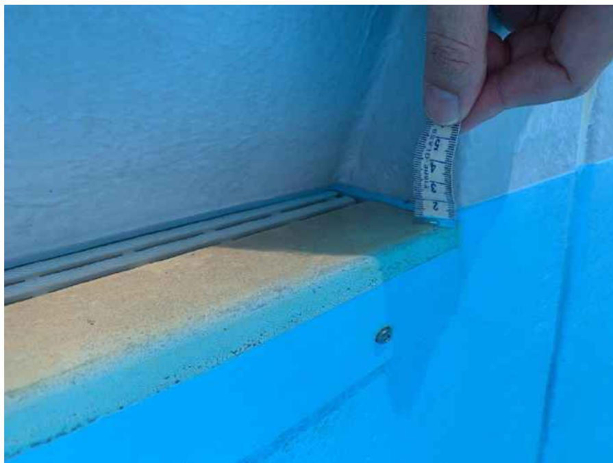
Figure 7: Scum Gutter in Lap Pool
