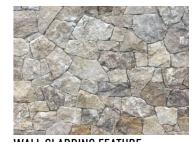
WALL CLADDING FEATURE EXTERIOR STONE VINEER FIXED TO BLOCKWORK WALL COLOUR: NATURAL WEATHERED EDGE
