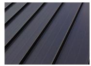
**ROOF CLADDING** STANDING SEAM METAL ROOF SHEETING, RIB HEIGHT 44mm, TRAY WIDTH 445mm. COLOUR: MONUMENT, COLORBOND
