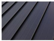
**ROOF CLADDING** STANDING SEAM METAL ROOF SHEETING, RIB HEIGHT 44mm, TRAY WIDTH 445mm. COLOUR: MONUMENT, COLORBOND
