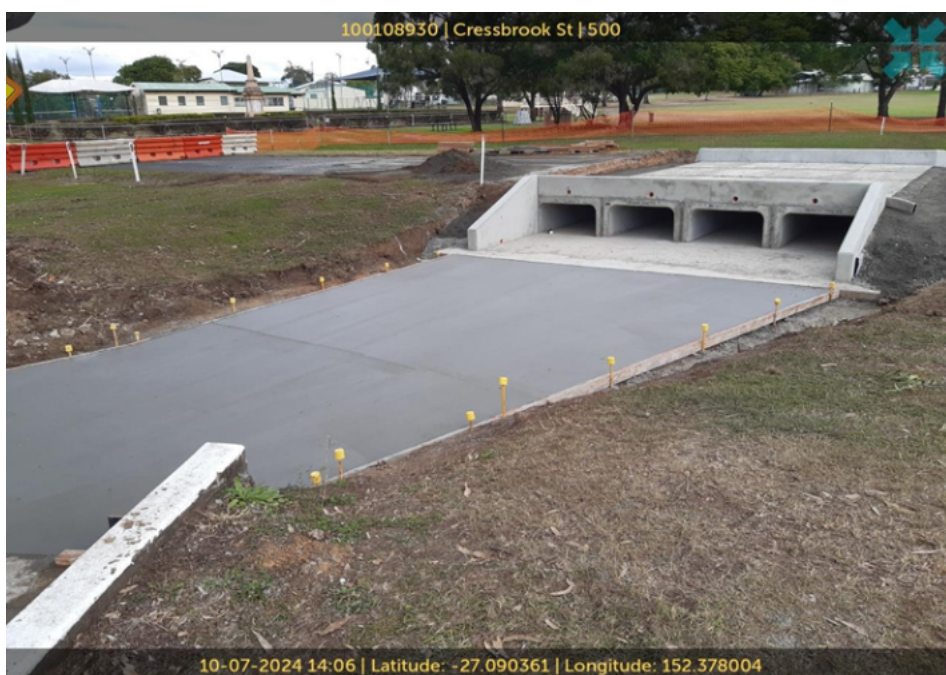
Cressbrook Street, Toogoolawah – replacement of three 1200mm culverts; rehabilitate road section with asphalt overlay.
