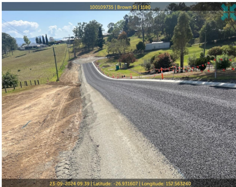
Brown Street, Kilcoy - provision of turnaround area for rubbish trucks and larger vehicles and also kerb and channel.
