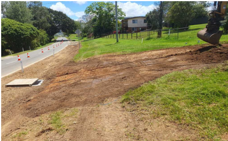
Kilcoy Murgon Road, Kilcoy - extension of underground drainage from Wade Street / Kennedy Street intersection.
