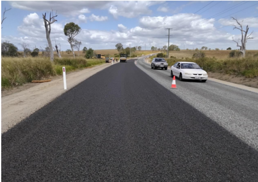
Brisbane Valley Highway – pavement Stabilisation. Funding: 100% Department of Transport and Main Roads
