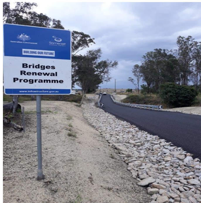
Tetzlaffs Bridge - completed Drainage Works
