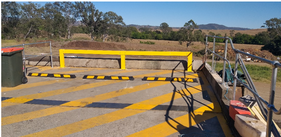
Heavy yellow safety rail installed at Kilcoy transfer station
