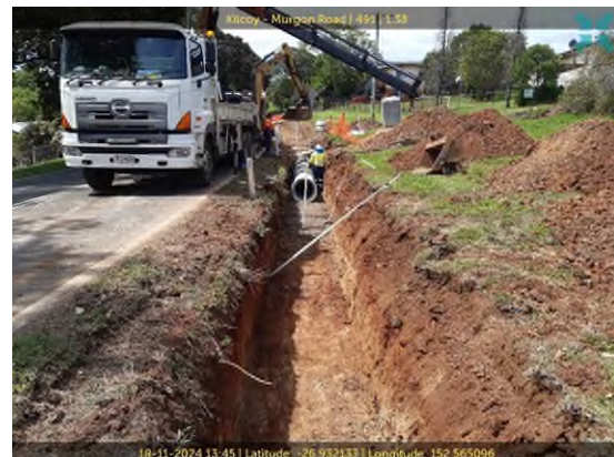
Kilcoy-Murgon Rd / Kennedy St, Kilcoy - extension of underground drainage –
