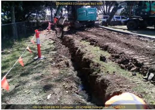
Kilcoy-Murgon Rd / Kennedy St, Kilcoy - extension of underground drainage –
