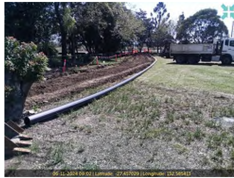
Kilcoy-Murgon Rd / Kennedy St, Kilcoy - extension of underground drainage –
