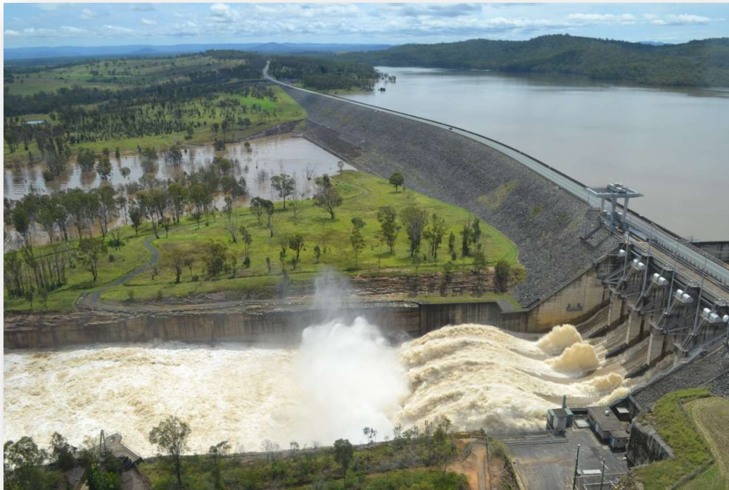
Figure 6: Wivenhoe Dam Release
