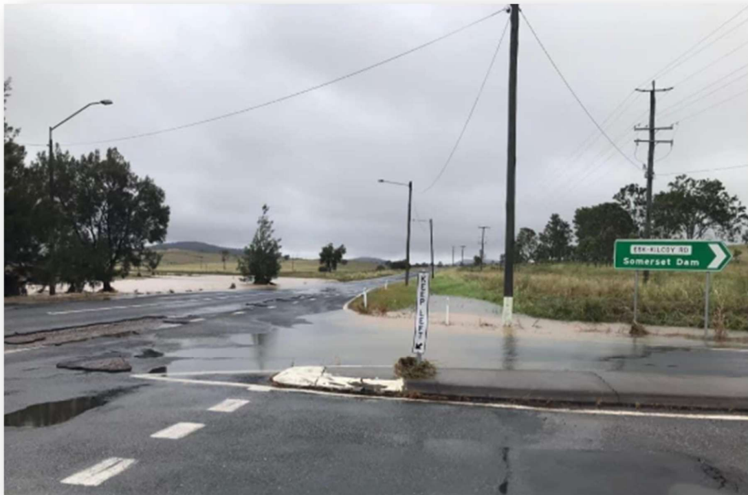
Figure 8. Flooding across Esk Kilcoy Road during the Feb-March 2022 Severe Weather Event
